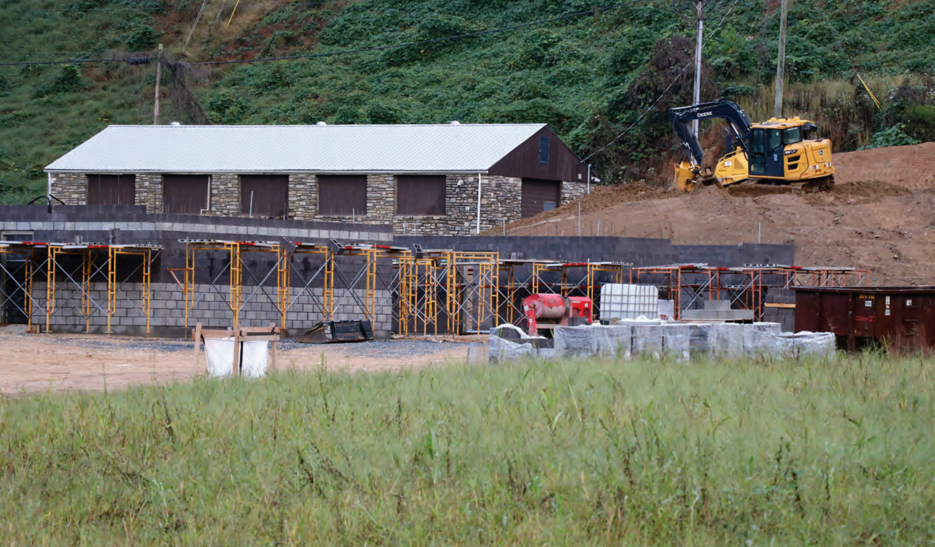
Progress is being made on the restroom facility at the new Cherokee Cultural Grounds as seen in this photo taken on the morning of Wednesday, Sept. 23. (SCOTT MCKIE B.P./One Feather photos)
