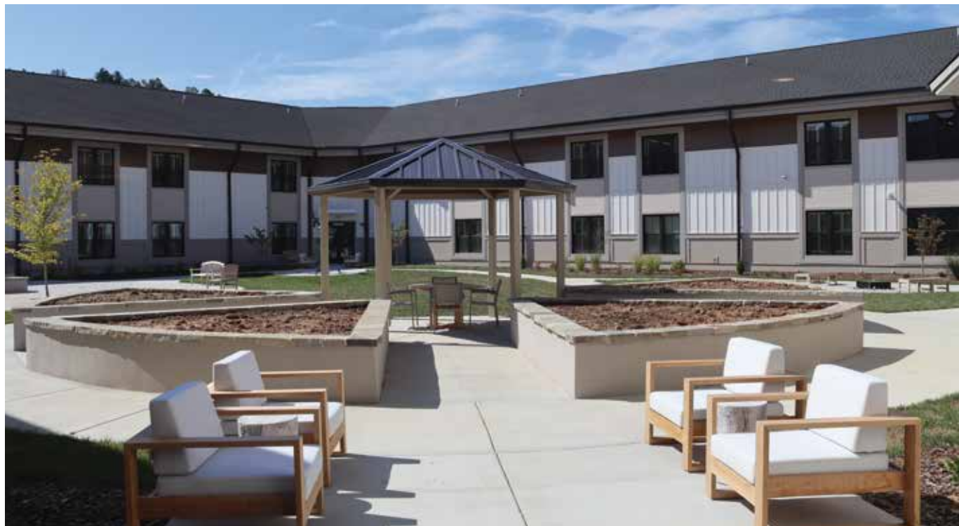
An outdoor space inside the new Tsali Care Center.
