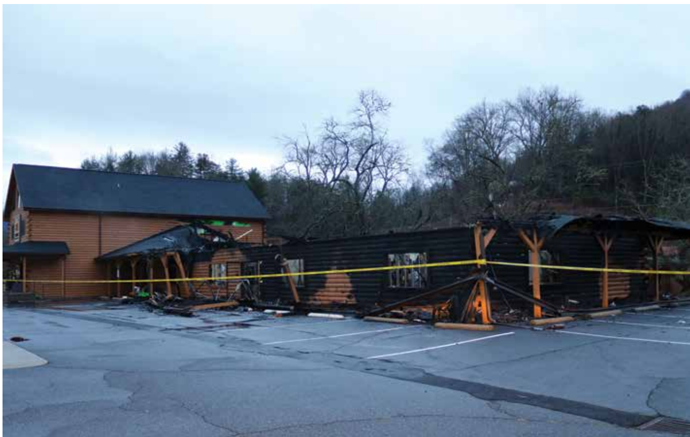
The Kituwah, LLC building burned in a fire on the morning of Thursday, Dec. 15. Cherokee Fire Dept. officials noted they were dispatched to the scene at 1:55 a.m. and, joined by crews from Bryson City, Qualla, Maggie Valley, and Savanna, extinguished the fire. They note that the cause is under investigation. The adjacent Kituwah Global Government Group, LLC building received slight fire and water damage. (SCOTT MCKIE B.P./One Feather photos)
