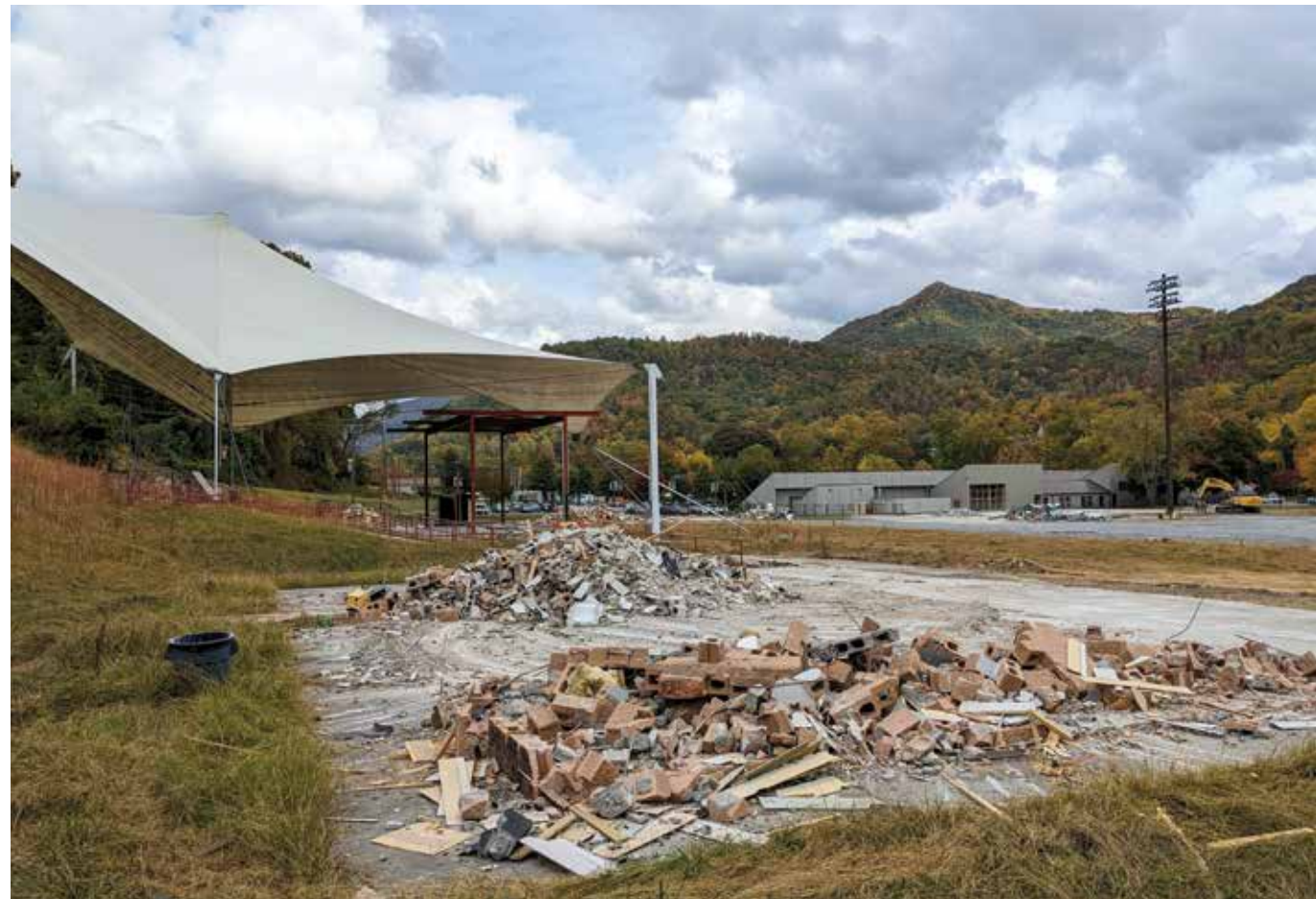
A photo, taken on the afternoon of Thursday, Oct. 13, shows the current demolition going on at the Cherokee Indian Fairgrounds. (ROBERT JUMPER/One Feather photo)
