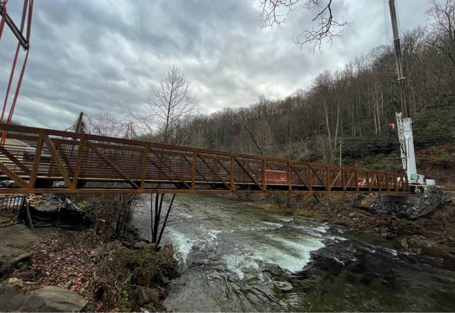
The bridge is now in place, and they can begin work on affixing the sewer line over the next two months.
