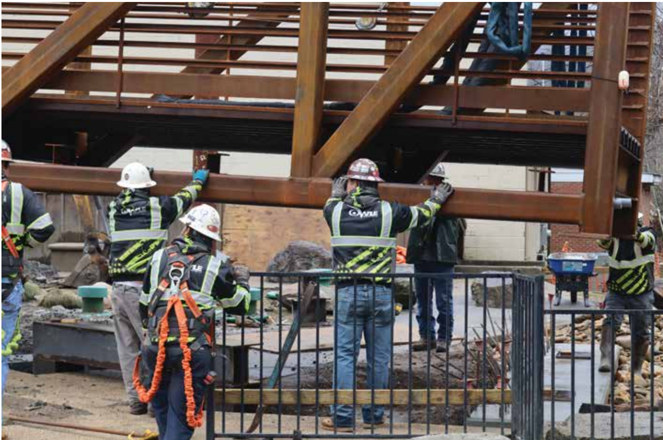
The entire crew for Owle Construction was on site for the bridge setting on Tuesday, Feb. 22. Workers had the brace the 90,000-pound bridge from swinging during the early stages. (JONAH LOSSIAH/One Feather photos)
