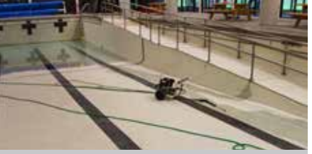
Cherokee Fitness Complex getting some renovations
