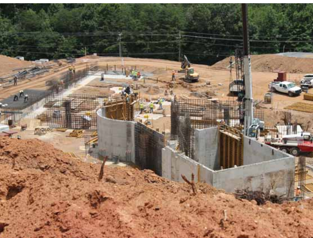
This photo, taken from above the main construction area, shows the concrete and steel being installed that will comprise the basement of the facility.
