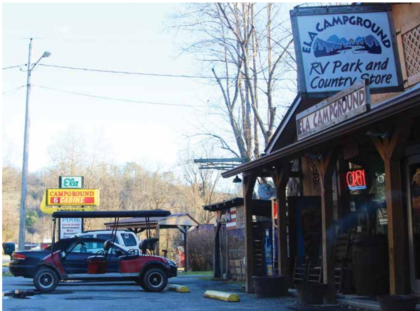
Kituwah LLC is in the process of remodeling the store and other facilities at Ela Campground & RV Park.
