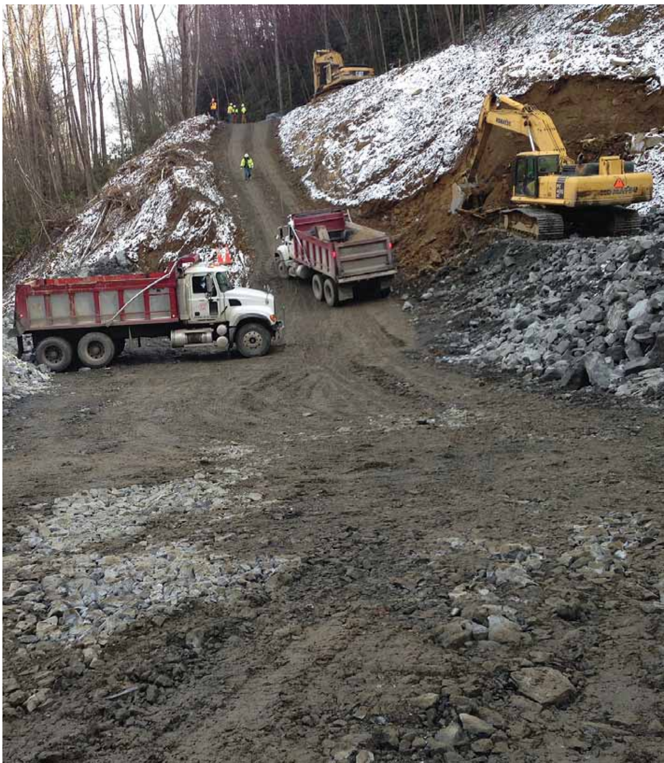
APAC—Atlantic, Harrison Division recently completed Phase 1 of the reconstruction project by developing an access road to the slide area, removing debris, and stabilizing the slope above the work area.
