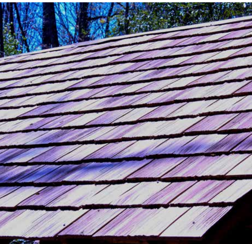
NEW TOP: Many buildings throughout the Village received a new roof of wooden shingles.
