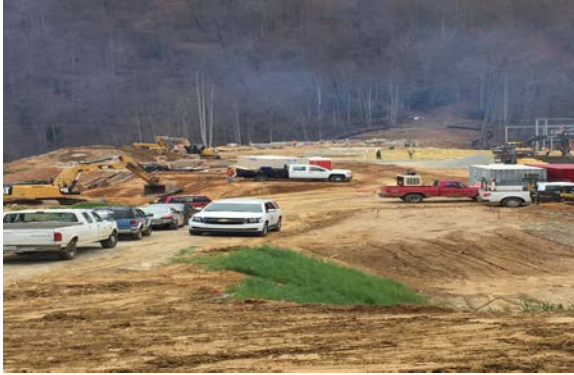
Construction of new Rehab Center
