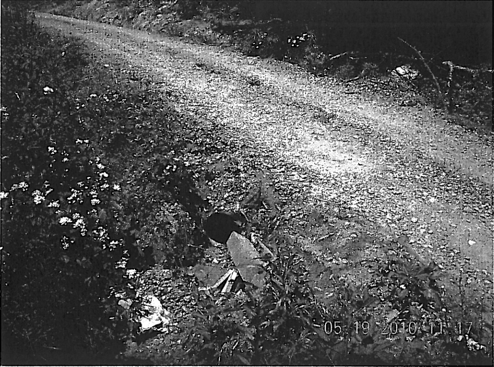
Picture showing location of single cross drainage
