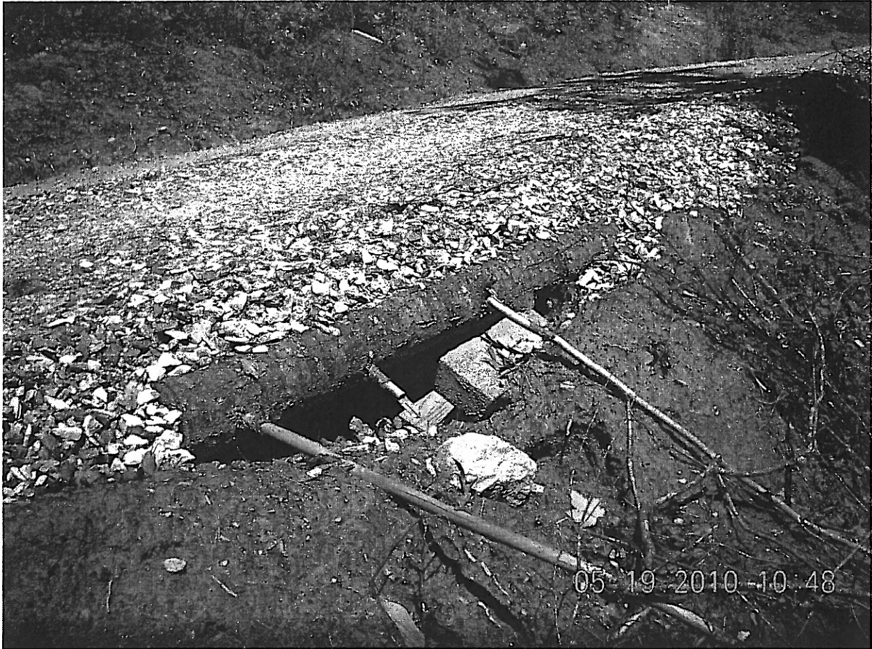
Homeowners attempt to stop erosion.
