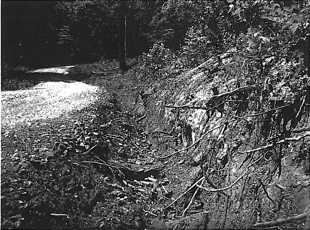
Pictures showing vertical sided ditch along
