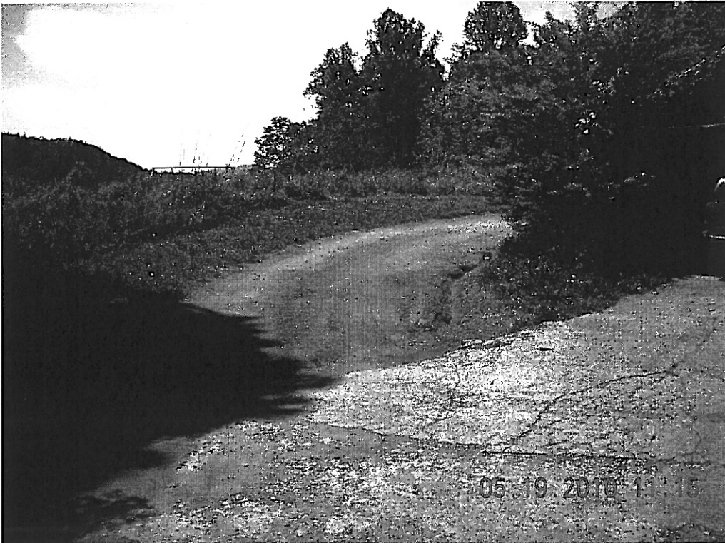
Beginning of driveway, note erosion of driving surface due to lack of
